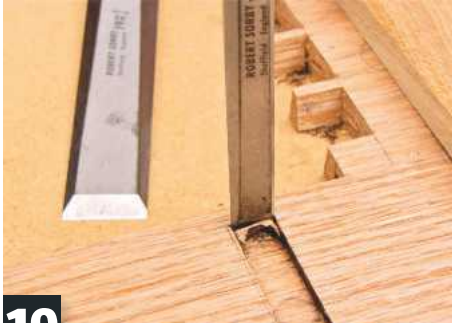
19 Housings are stopped 5mm below top edges. Square rounded ends neatly with chisel
